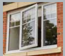
INSTALL NEW WINDOWS
